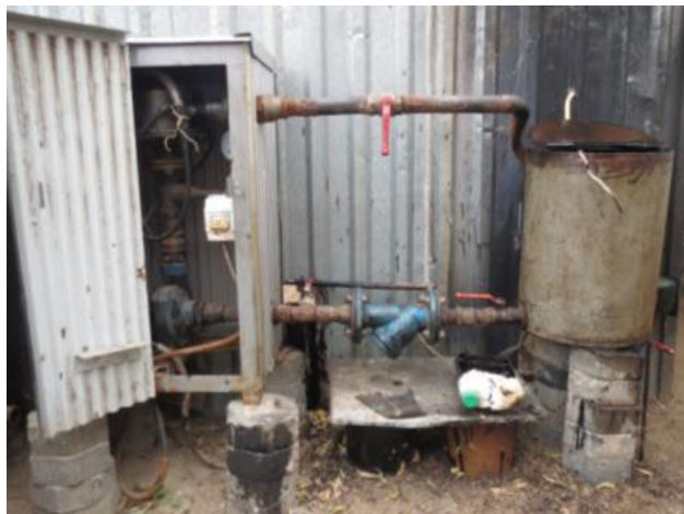
Figure 2 – Dispersion system for watered fuel oil
