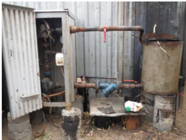
Figure 2 – Dispersion system for watered fuel oil
